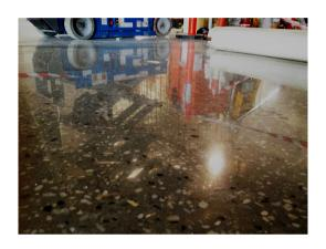
As part of the Formula Worx range of floor treatment products, TBP is a uniquely formulated concrete hardening & densifying agent. Surface harness can be improved dramatically within 24 hours, providing long term increases in strength, abrasion and stain resistance of concrete floors.
